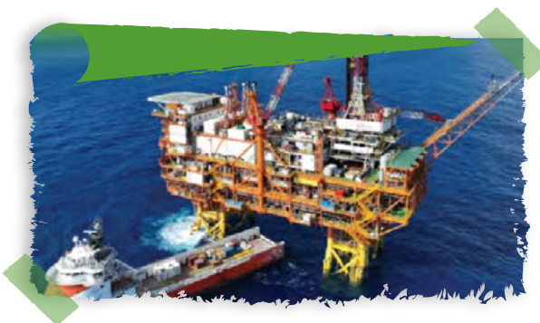
China's First Offshore CCUS Project Commissioned
