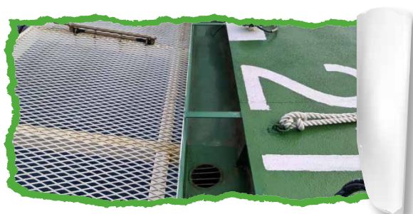
Rainwater Collection Troughs on Helicopter Platform Deck
